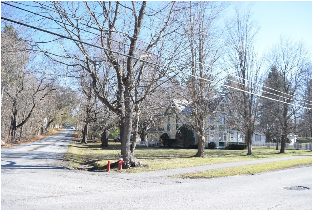
Photo 9. View of Hawks Avenue (left) looking from the intersection with Bank Street. Note the fire hydrant in the foreground. A close-up view is in Photo 10. View facing east-northeast.
