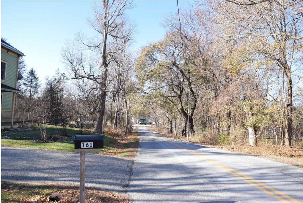
Photo 8. View along Hawks Avenue. Note the grass drainage ditch and elevated yard, indicating the area of the road and shoulder was graded. View facing west-southwest.
