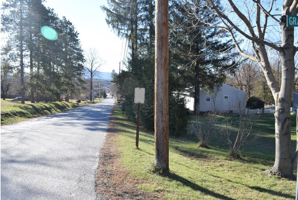
Photo 2. View along Grandview Street. Note the rise of the landform to the left of the road and the downward slope from the right shoulder of the road indicating significant grading occurred during the construction of the roadbed. View facing south.
