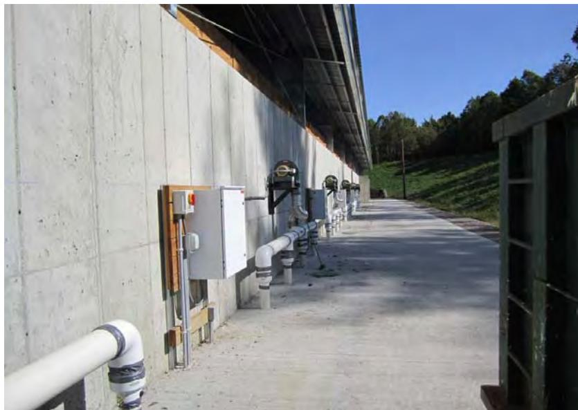
*Figure 7: Blowers in area D of figure 1. These blowers are fairly large (nominally 1+ HP) and*
