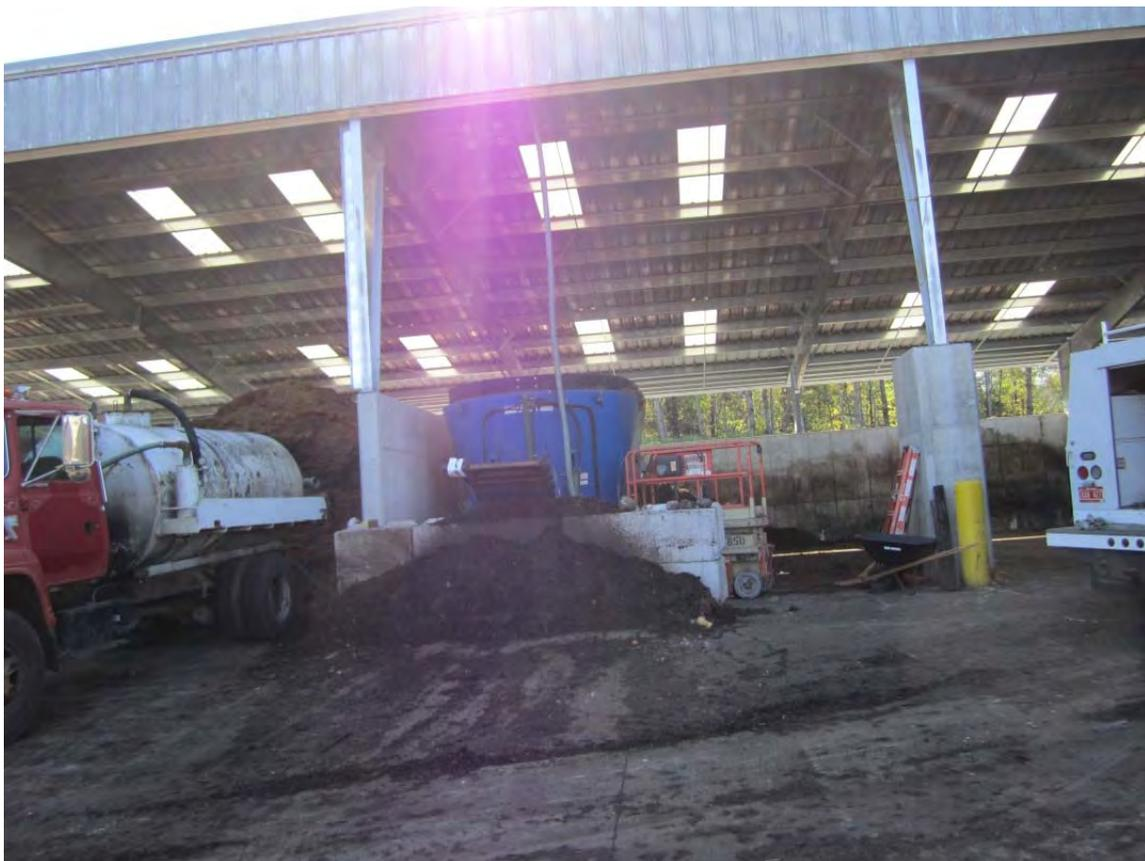
*Figure 5: Shed for active phase 1 composting. The blue vessel in the center is a blender where the mixture of food waste, horse manure and water is created with the desired carbon/nitrogen ratio and*
