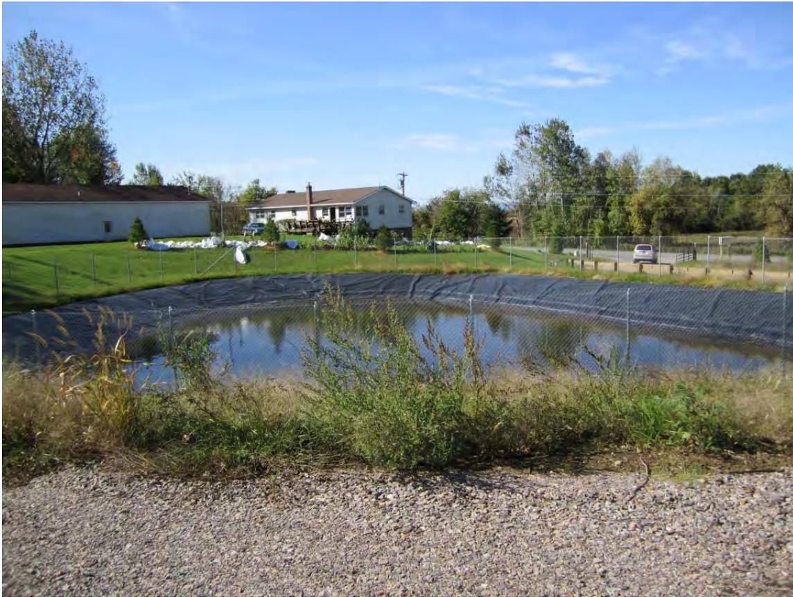
*Figure 8: Lined pond for collecting leachates (and rain water) during active phase 2 composting. The water in this pond is almost free of contamination. The residence on the other side of the pond labeled L in figure 1 is owned by CSWD and is rented at a reduced rate.*
